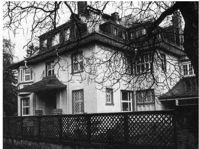
5 Villa in Wiesbaden-Biebrich 5 Villa in Wiesbaden-Biebrich
